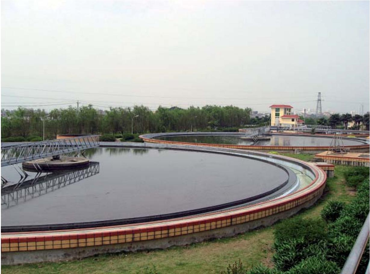
The project is located in Dongdun Village and Xianying Village, the combined area of Chengxiang District and Hanjiang District of Putian City, Fujian Province, the PRC. It involved the design and construction of a wastewater treatment facility with a wastewater treatment capacity of 80,000 tonnes per day in the short term and 160,000 tonnes per day in the long term. The treatment process adopts the improved oxidation ditch technique.
