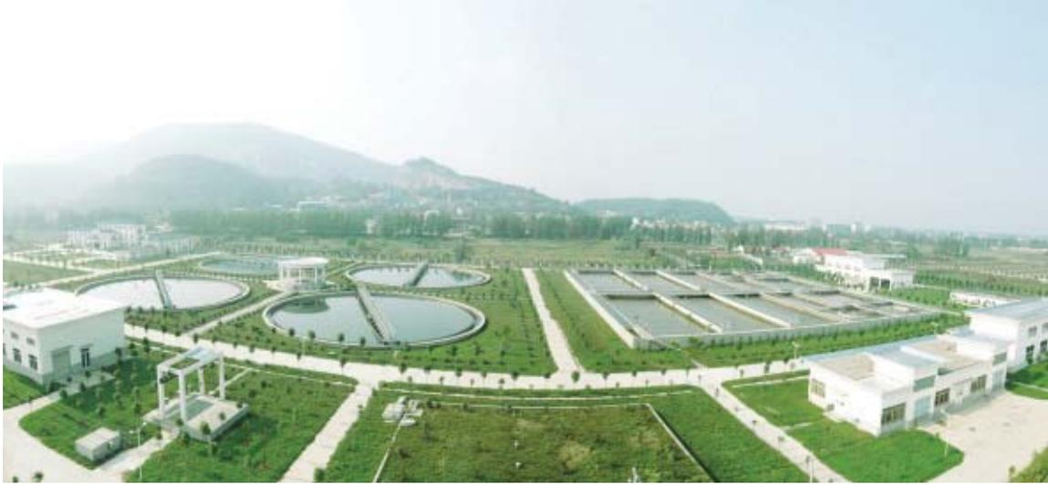
The project, located in Xiangcheng District of Xiangfan City, Hubei Province, involved the design and construction of a wastewater treatment facility with a wastewater treatment capacity of 100,000 tonnes per day. The treatment process adopts the A<sup>2</sup>/O pre-denitrification technique.
