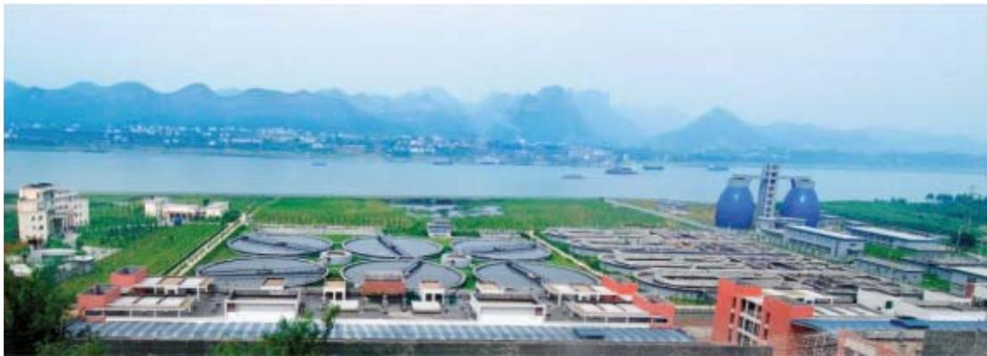
The project involved the design and construction of a 440,000 tonnes/day water treatment facility, a 200,000 tonnes/day wastewater treatment facility and laying part of the pipeline network system of Yichang City, Hubei Province. The water treatment plant provides tap water for the entire city of Yichang, which has a population of more than 4 million.
